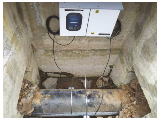
Installation of Clamp-On Type Ultrasonic Flow Meter
