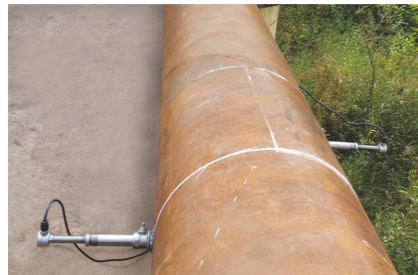
Installation of Insertion Type Ultrasonic Flow Meter
